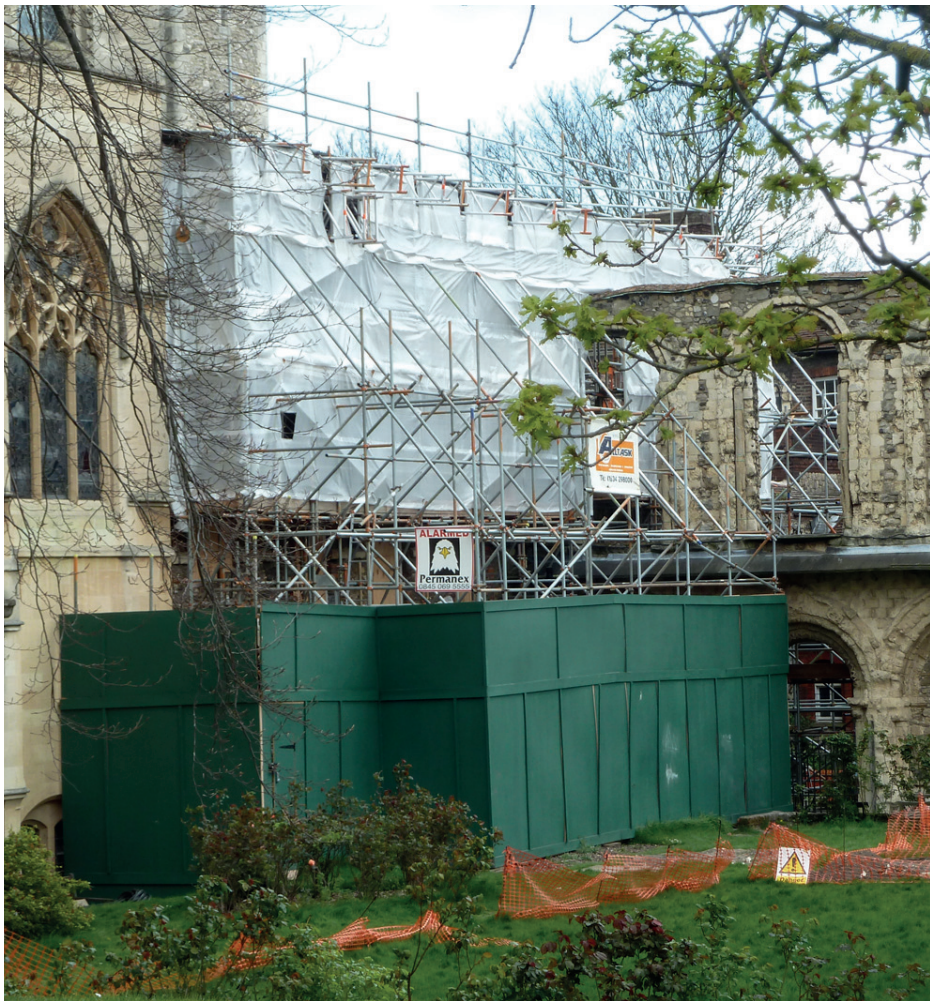
Works in progress on the Chapter House
