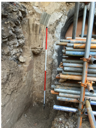
The corbel and springing of the 14th-century vaulted passage, with the rendered west wall of the 12th-century Chapter House to the left. The gravel and rubble core above this is probably part of the 14th-century work
