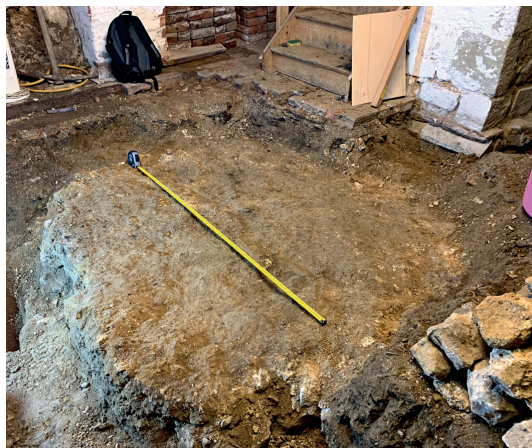
Figure 6: Foundation in the western basement.
