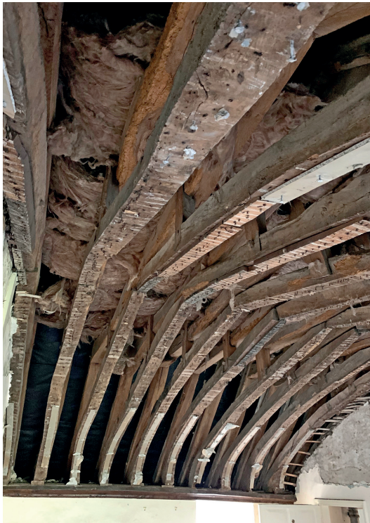
Figure 8: Medieval roof over the eastern second-floor bedroom.
