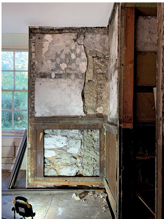
Figure 7: Blocked medieval door in the eastern ground-floor living room.
