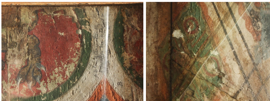
Fig 3. Raking light details of lifting and flaking paint
