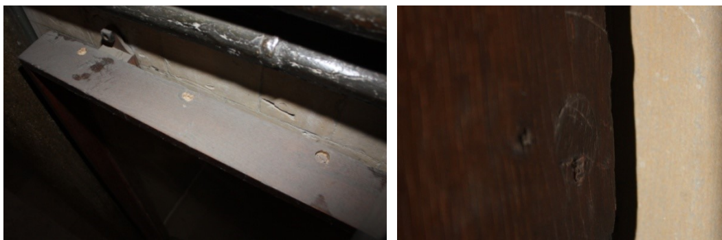
Fig 2. Countersunk screws on the side and bottom are covered by oak plugs.
