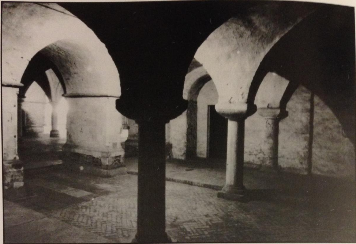
The western end of the crypt showing evidence of Gundulf's work
